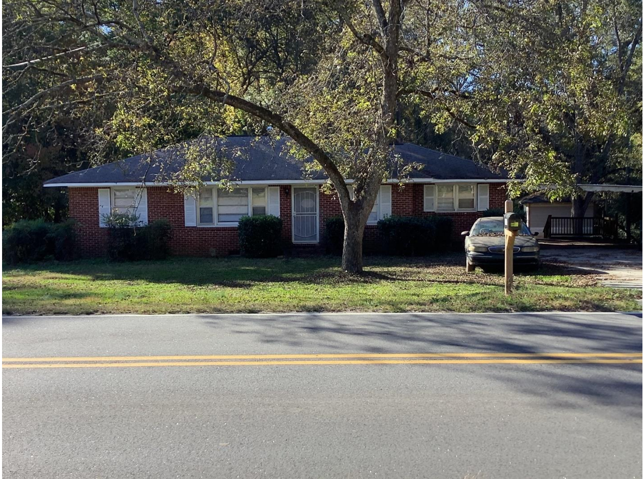
Figure 84: 1308 South Madison Avenue (GNAHRGIS #283765); example of the Plain Style
