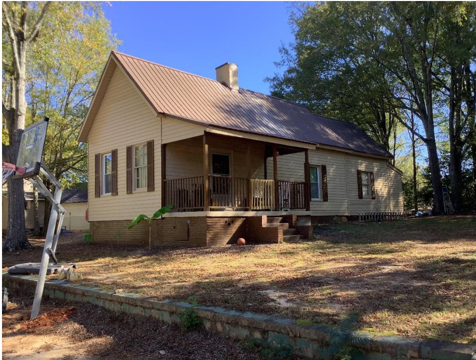
Figure 60: 122 Norris Street (GNAHRGIS #64833); example of an Unidentified House Type
