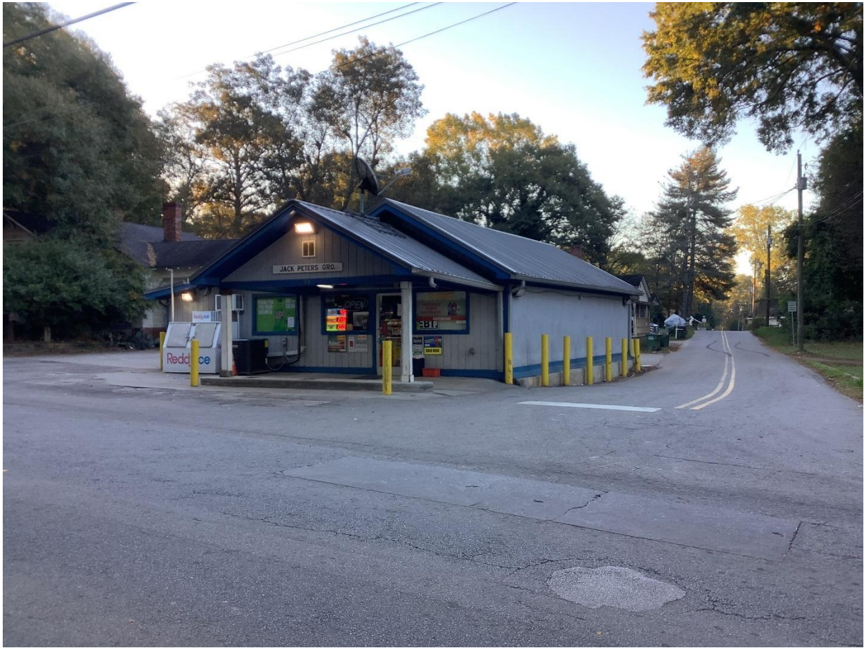
Figure 70: 800 East Church Street (GNAHRGIS #282948); example of a Gas/Service Station; the original gas pumps have been removed
