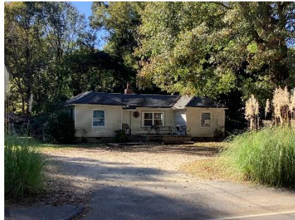
Figure 52: 1218 South Madison Avenue (GNAHRGIS #283745); example of a Courtyard Ranch
