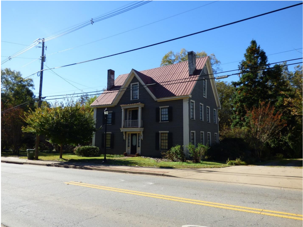
Figure 42: 432 South Broad Street (GNAHRGIS #283251); an example of a Georgian House
