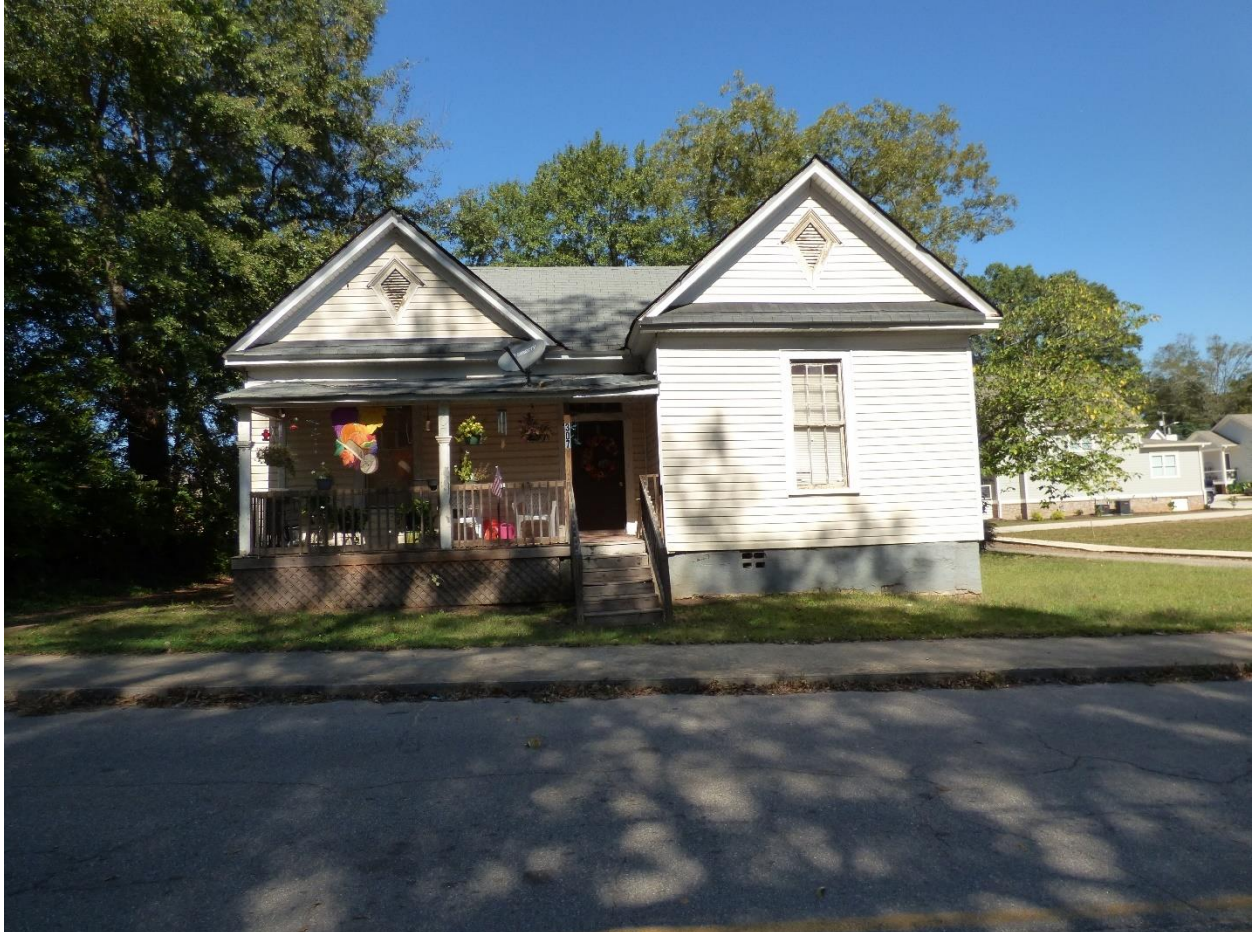
Figure 46: 307 Davis Street (GNAHRGIS #281358); an example of a New South Cottage
