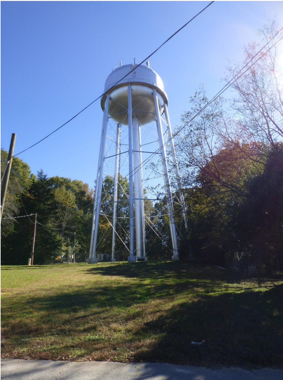
Figure 73: 110 Norris Street (GNAHRGIS #283256); example of a Water Tower
