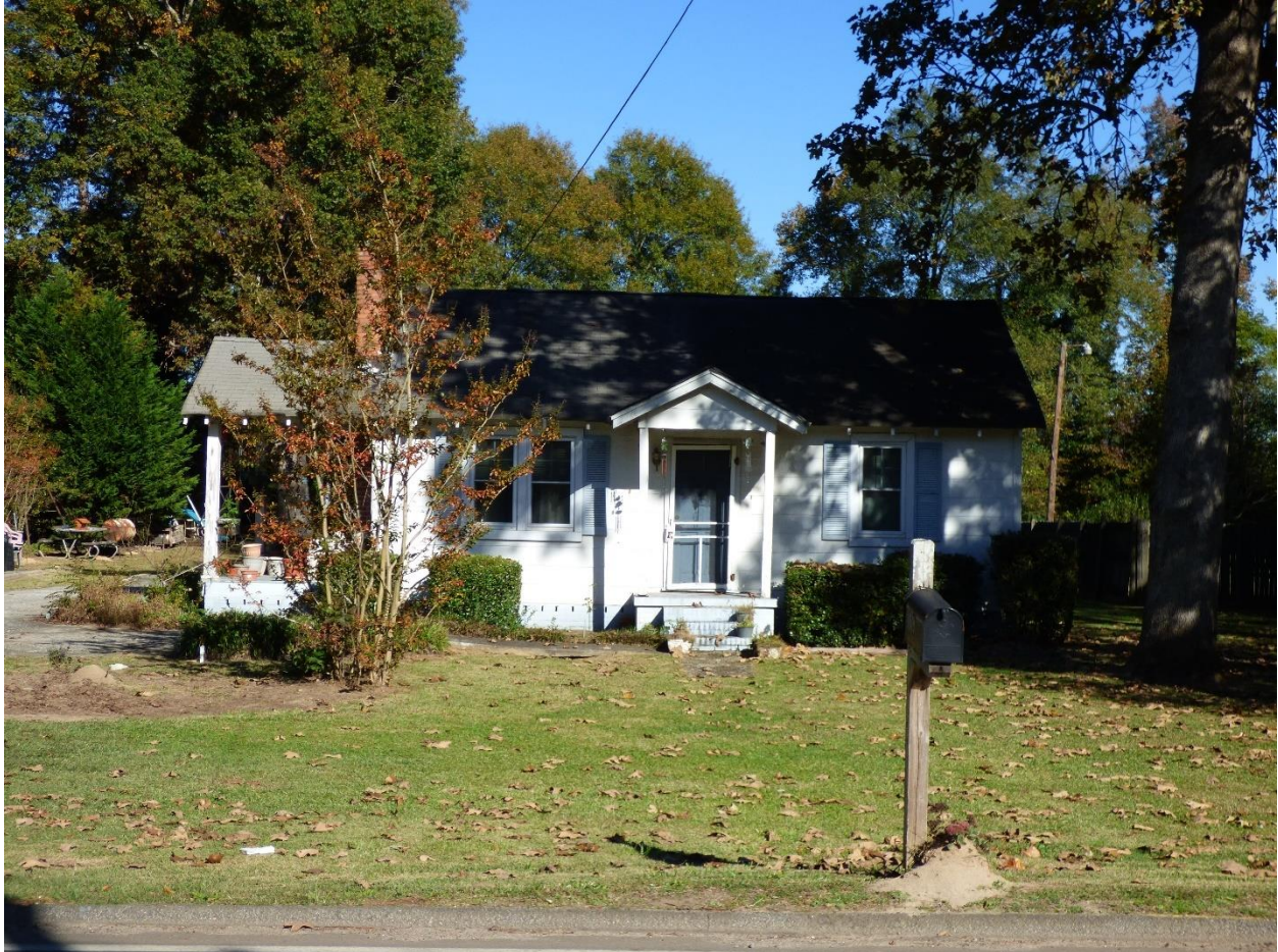
Figure 32: 1019 South Madison Avenue (GNAHRGIS #283718); an example of an American Small House
