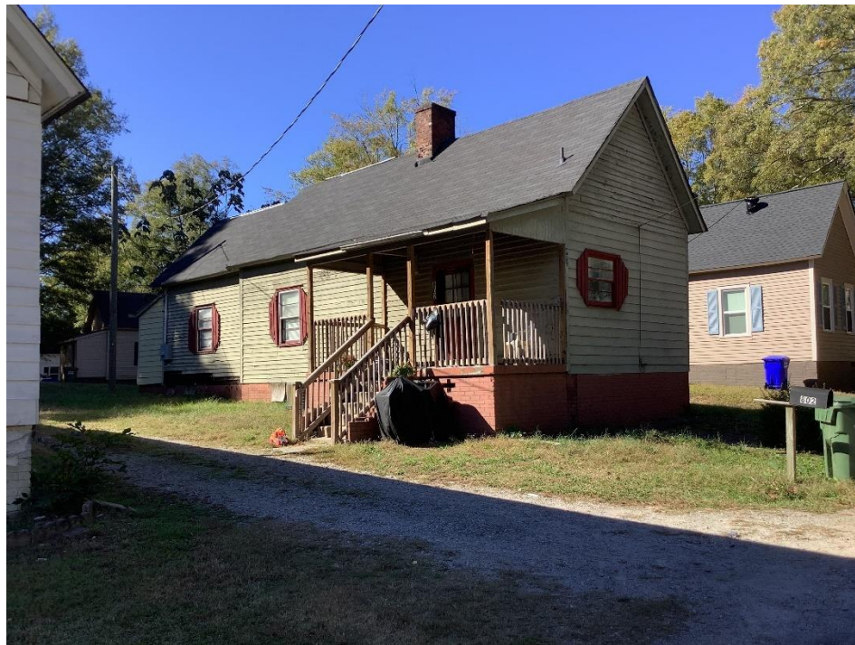
Figure 61: 802 Radford Street (GNAHRGIS #283223); example of an Unidentified House Type
