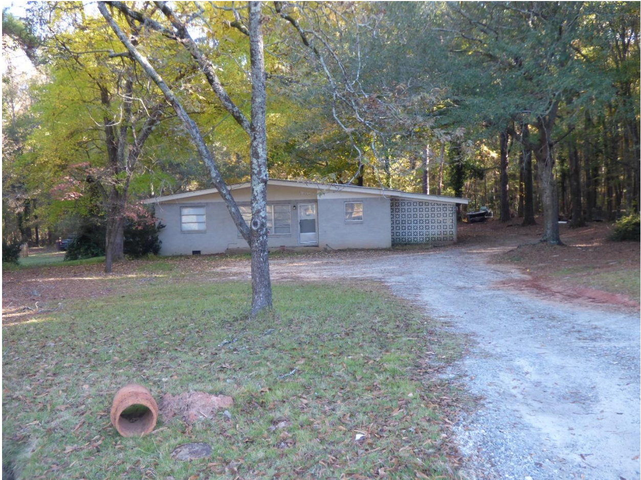
Figure 77: 1445 South Broad Street (GNAHRGIS #283307); example of the Contemporary, “Eichleresque” style
