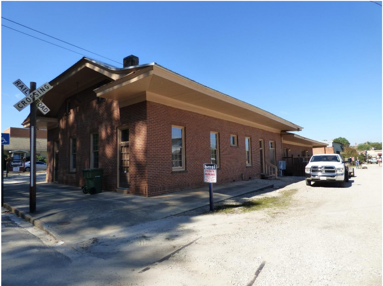
Figure 69: 115 Davis Street (GNAHRGIS #281353); example of a Train Depot
