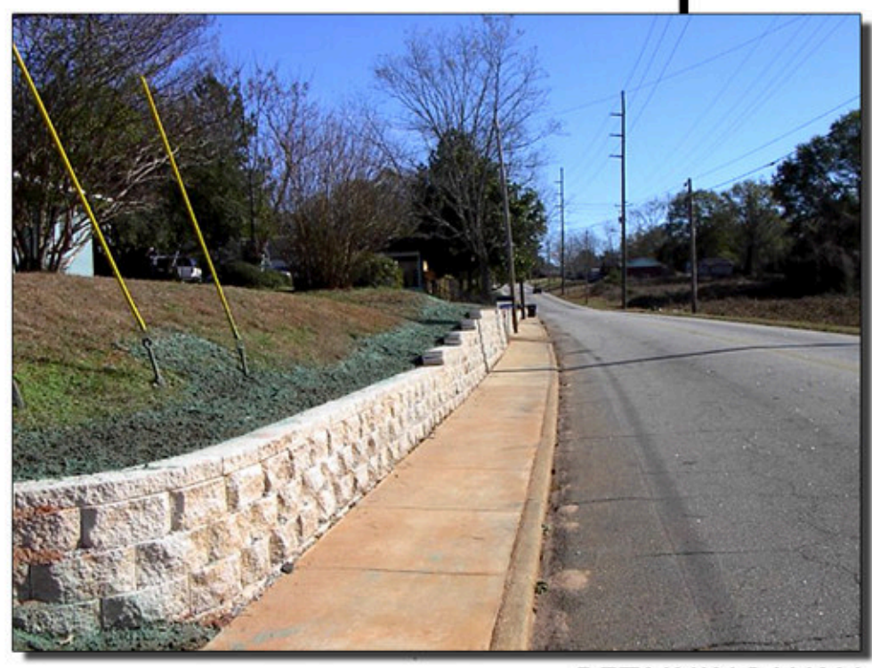
RETAINING WALL NEWNAN, GA
