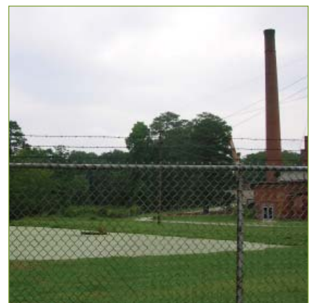
A retaining pond in front of Avondale Mill could become an open space with redevelopment
