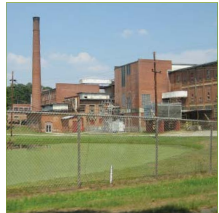
The redevelopment of Avondale Mills could include a multi-use trail
