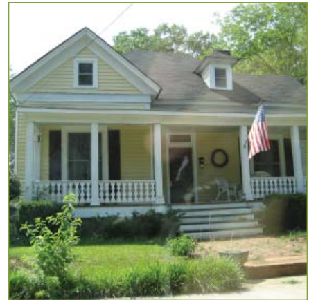
This home is one of many examples of residential development in established neighborhoods
