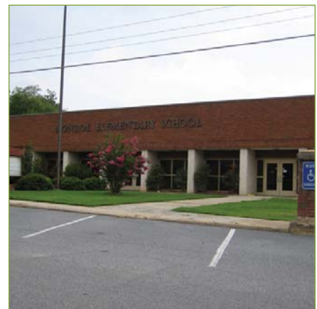
The Monroe Elementary School could be converted into a use such as a community center
