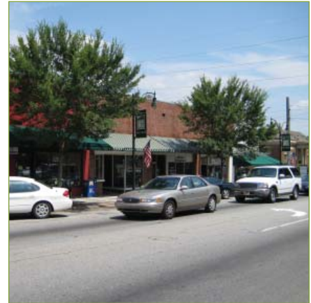
Small lots contain small building patterns, placed at the front of the parcel to meet the sidewalk
