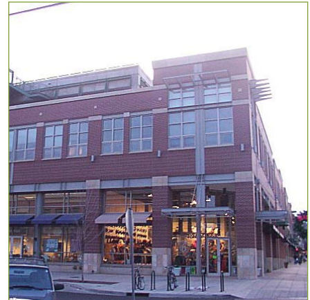
This public parking deck in Boulder, CO, is lined with retail and offices and fits in with its downtown
