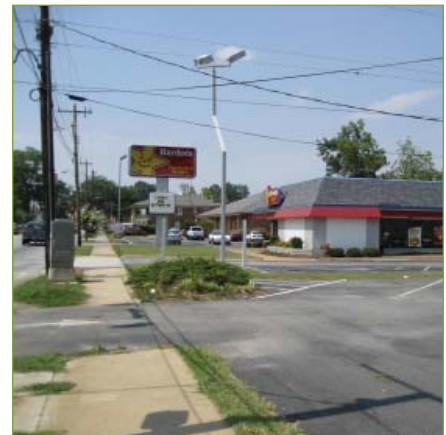
Medium to large parcels easily accommodate automobile oriented uses
