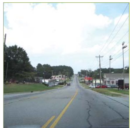
SR 10 (Spring Street) includes a center turn lane east of downtown
