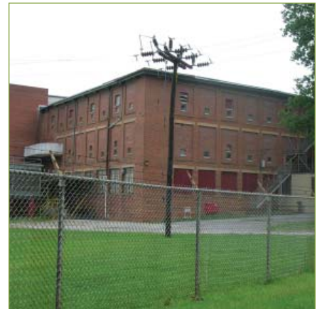
Historic Mill structures are often ideal for adaptive reuse into residential units or other useable space
