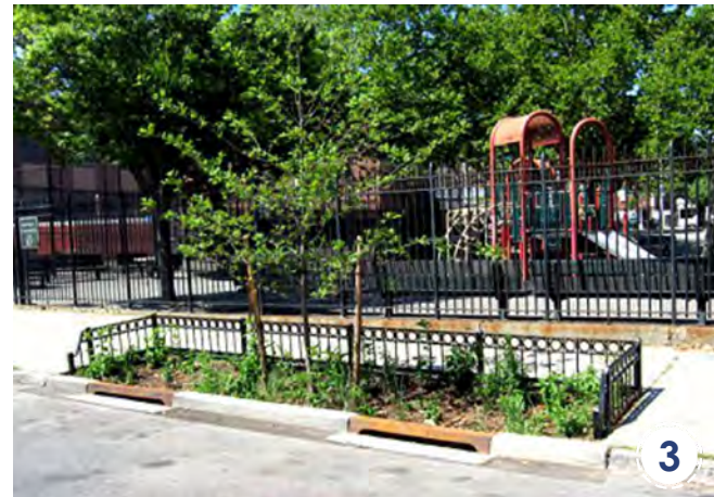
3 Appropriate example of a stormwater planter with tree (with or without fencing)
