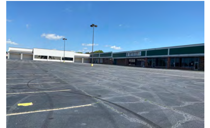
View of Existing Building Looking North
