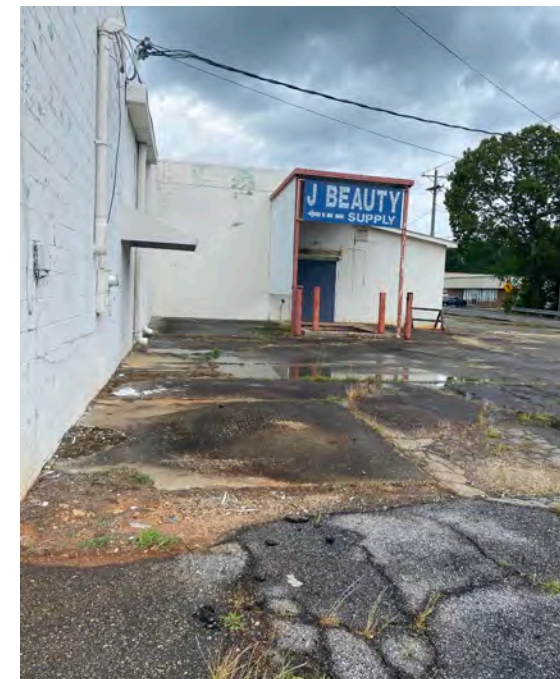
View of Rear Side of Existing Building
