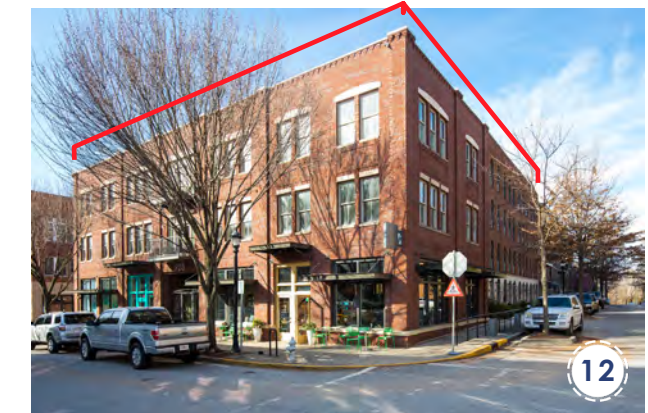
Example of a building lacking differentiation from bay to bay
