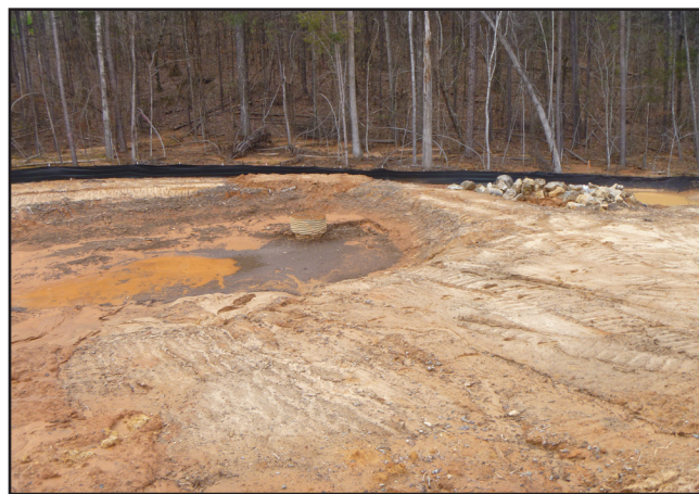
Figure 2.1 - Energy of falling raindrops has detached and transported soil particles from unprotected areas.
