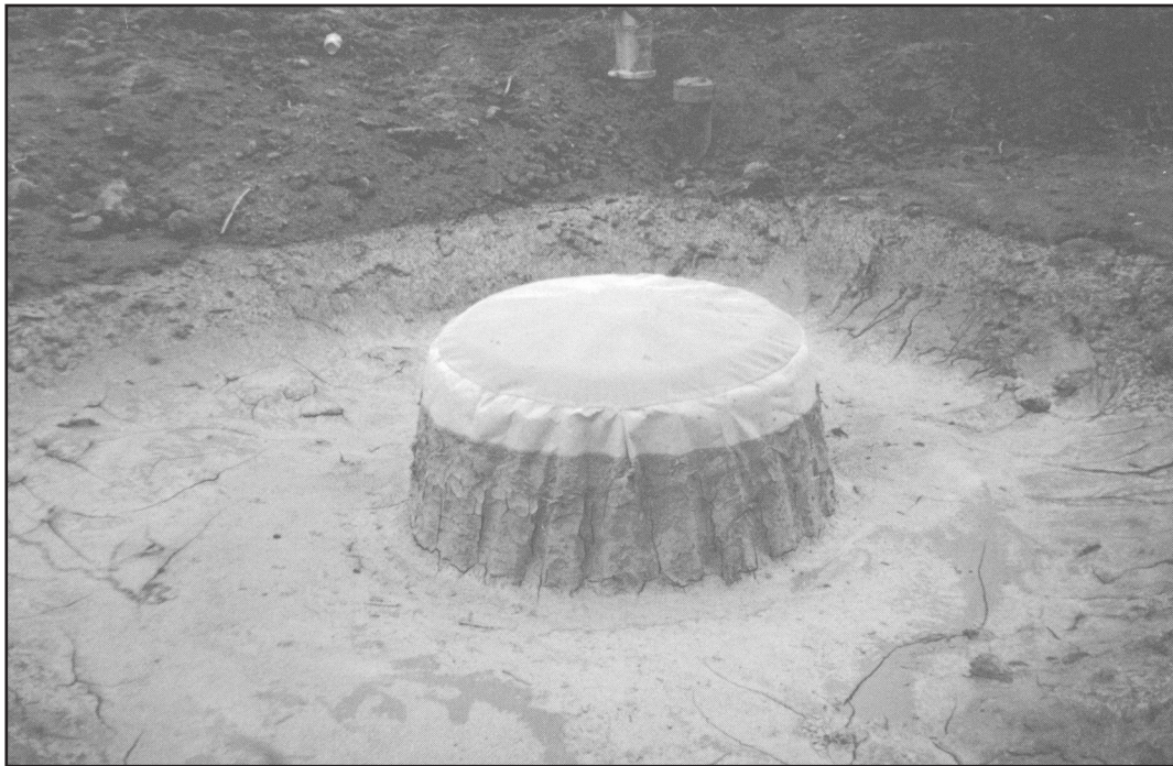
Figure 6-28.7 Equivalent Inlet Sediment Trap
