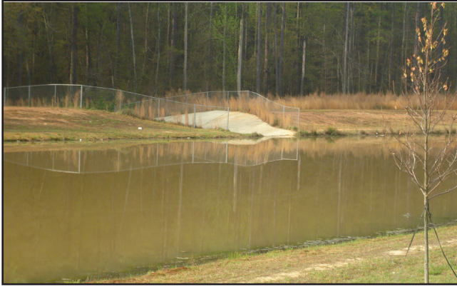
Figure 2-12. - A temporary sediment basin converted to a permanent pond enhances landscape.
