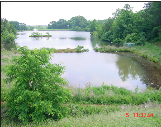
Post-construction conversion called for the creation of sediment forebay in this larger scale pond.
