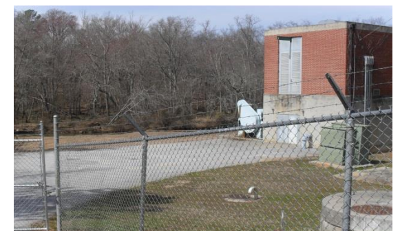
Alcovy River Pump Station
