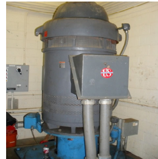
Verticle Turbine 5,500 GPM Delivers 3.82 MGD
