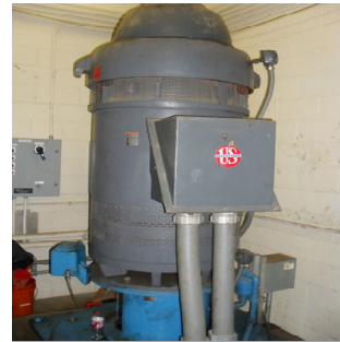
Verticle Turbine 5,500 GPM Delivers 3.82 MGD
