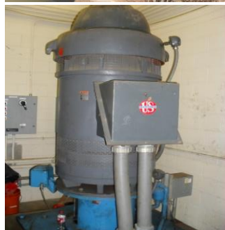
Verticle Turbine 5,500 GPM Delivers 3.82 MGD
